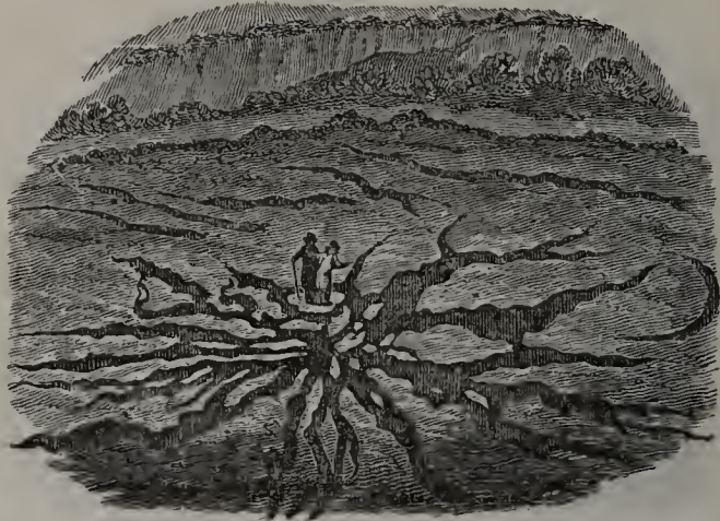
Fissures near Jerocarne, in Calabria, caused by the earthquake of 1783.)
